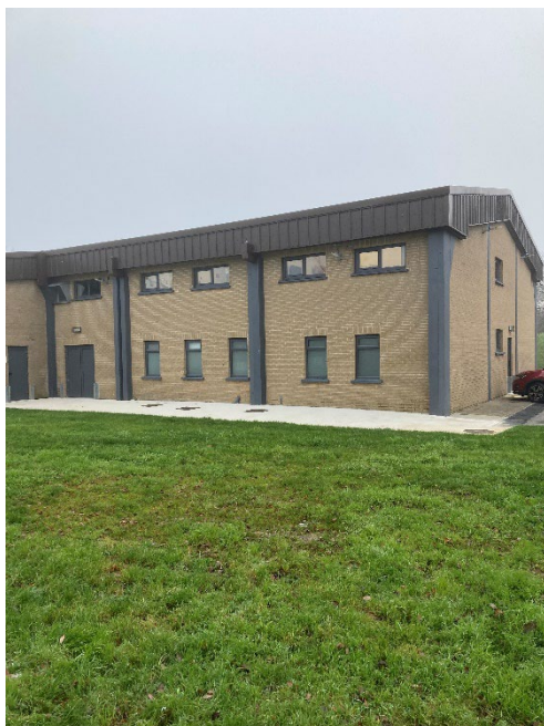
Rear Exterior building façade
