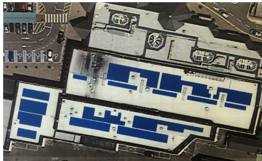
Figure 21 – Overhead view of the Solar panels on the roof of SuperValu
